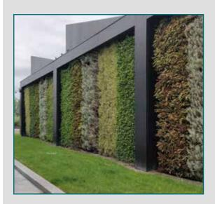
Living walls are wall-mounted growing systems. They can directly intercept precipitation, and utilise harvested rainwater, to attenuate peak flows and both improve quality and decrease quantity of surface water run-off.
