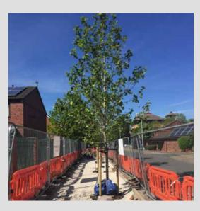
Tree-trenches with suspended pavement facilities can offer water storage, water-cycling and attenuation, and help reduce pollutants through filtration, absorption, microbial action and tree uptake.
