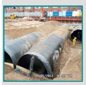
Underground structures with capacity to store water below ground.
