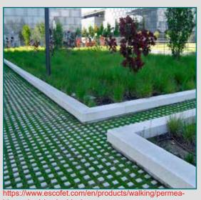
Pervious paving allows water to infiltrate its surface and flow through its construction layers. Water then either infiltrates into the soils below or collects into an outfall.
