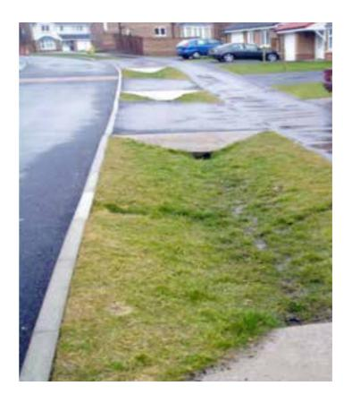
Image showing a grassed swale incorporated in a roadside verge
