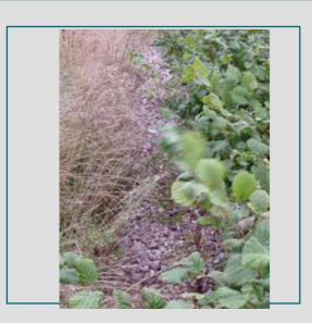
Gravel or rubble filled trench that creates subsurface storage for infiltration, or filtration of surface water runoff.
