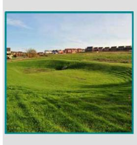
Vegetated depressions in the ground that have been designed to attenuate storm water flows by providing temporary storage. They can also help improve surface run-off quality as they offer some pollution removal due to settling of particulates.
