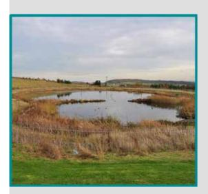
Retention ponds are structures that provide both retention and treatment of contaminated storm water run-off.
