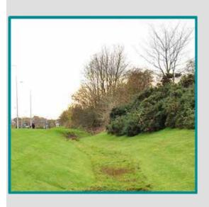
A vegetated shallow channel or depression designed to treat, filter, store and convey run-off.
